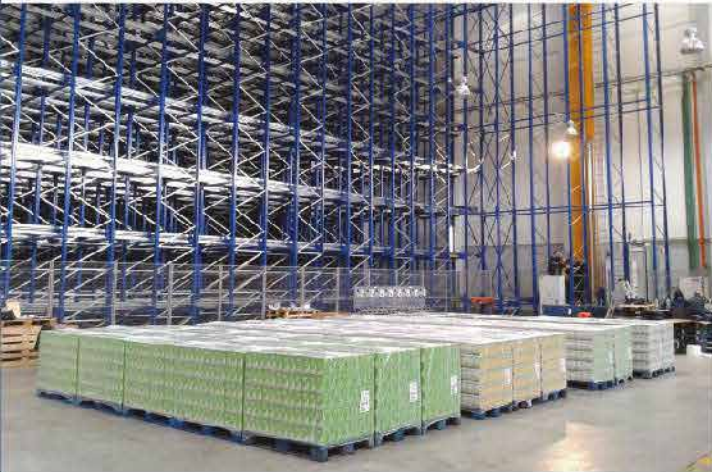
Satellite Storage System Using Automatic Pallet Crane
